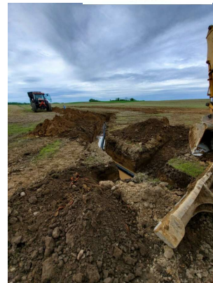
Field improvements (Picture: tiling)
